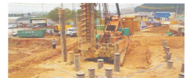
Foundation work with DTH hammer & bit
